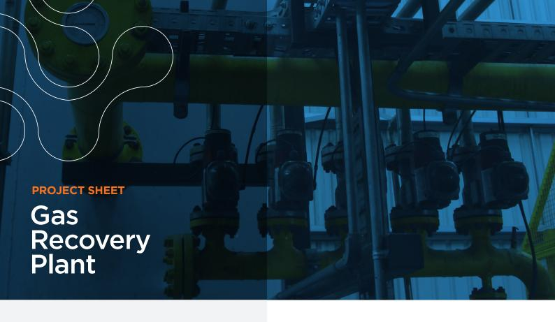
Carnot supported an Australian company with the complete design of a gas recovery system, which collects remnant gas from disused gas bottles and aerosol containers when they are crushed. Recycled bottles contain a variety of gas types and quantities that must be accommodated. The recovered gases are made available for use within the process plant for firing boilers.
